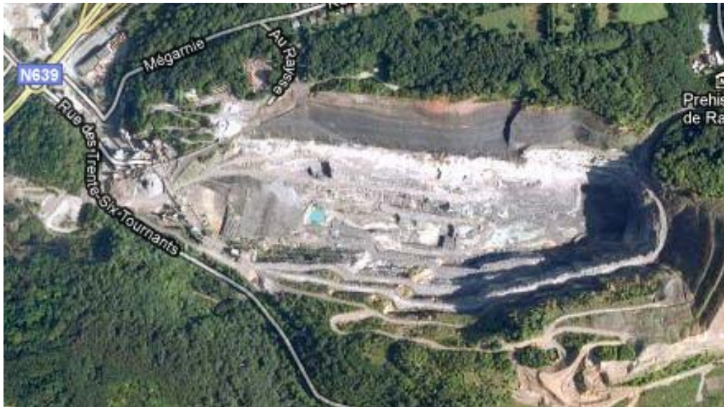
Fig. 3: aerial view of the mono-landfill of Prayon SA
