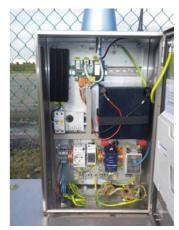
The **aerosol stations** (ZnS detector), of which there are 7 for measuring the <u>radioactivity of dusts</u> suspended in the air (aerosols and fine particles), which determine the <u>total alpha and total beta</u> radioactivity.
