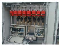
The collect of air dusts is realized by using pumps, air is passing through a filter which impacts dusts on a filter (photo on the left – automatic system).
