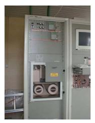
The photograph on the left shows the alpha/beta measuring unit with a view of the unreeling filter tape which collects the dusts and particles impacted when the air is pumped.
